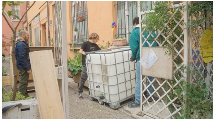
Figure 3 Rainwater collection tank being installed in Bologna. Source: ENEA
